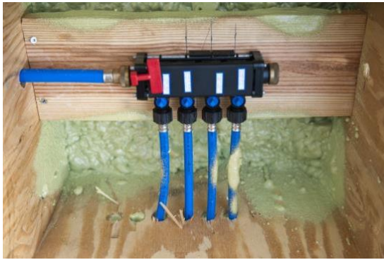
Figure 1 Manifold hot water system
