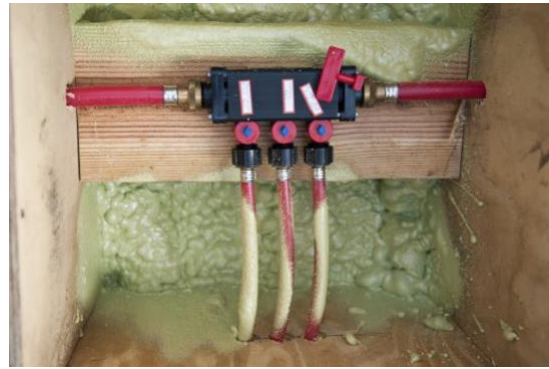
Figure 2 Manifold hot water system
