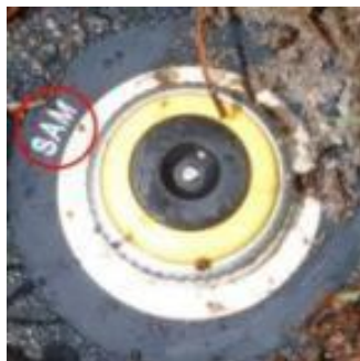
Figure 1 Photo shows “SAM” which stands for Seal-A-Matic check valve
