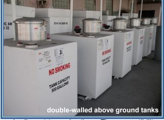
Many fluids should not be mixed or stored adjacent to each other. The compatibility of fluids is especially important to understand when the potential for adverse reactions exists, such as between oxidizers and flammables. In addition, materials are easier to manage and more cost effective to recycle when they are segregated.
